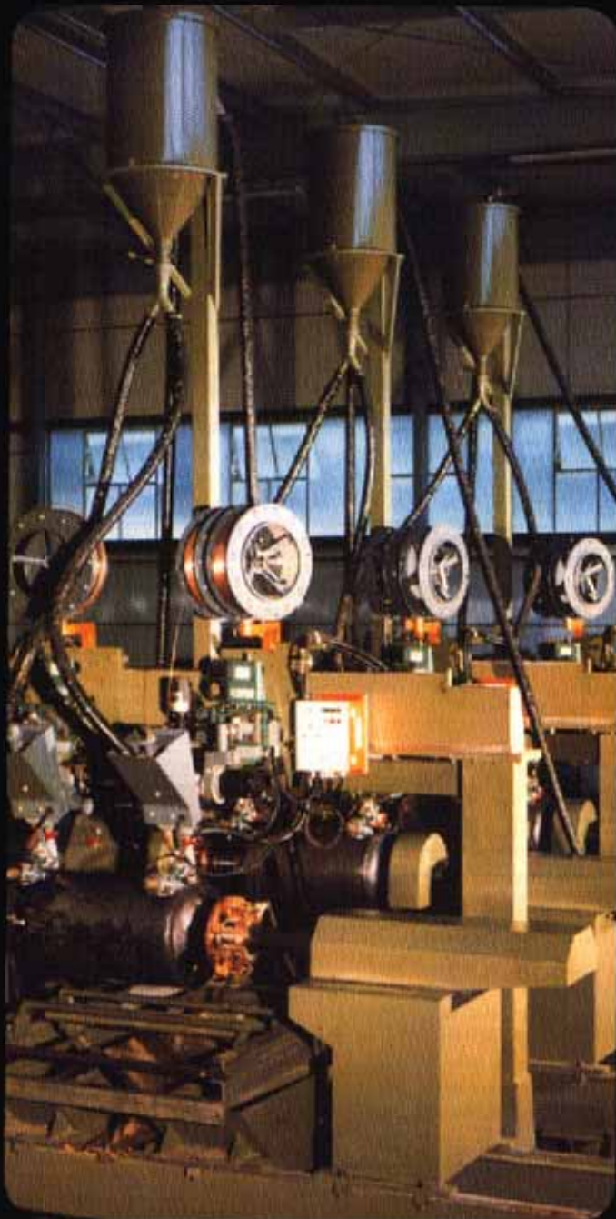
Primary separators are mounted high above the automatic welders, and at a distance from the vacuum source. Each separator serves two SAW flux hoppers.
